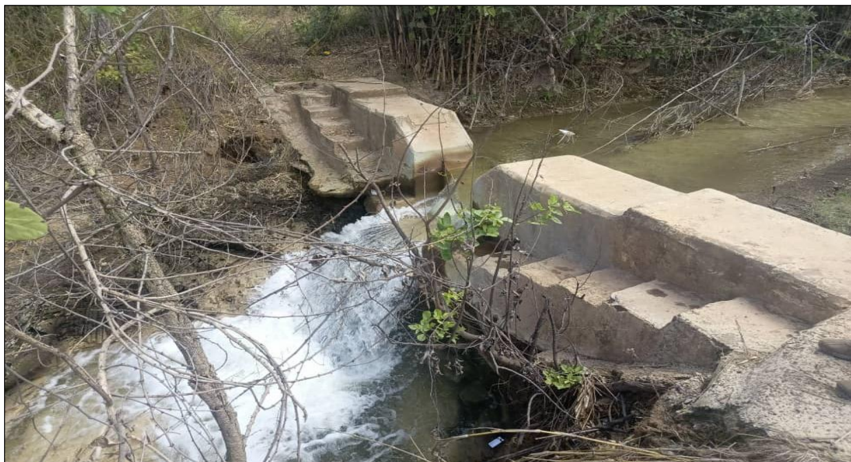
Figure 4-76: Photograph showing v-notch weir at the discharge from New Dam to Chambishi Stream
